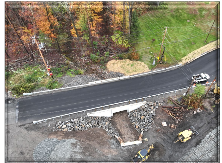
Precast Concrete Box Culverts over Tributary to Roaring Brook Creek
