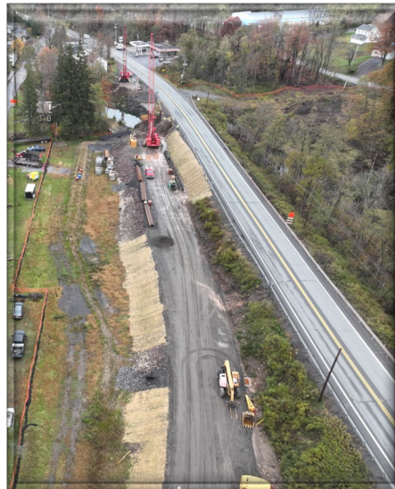
Temporary Bridge over Roaring Brook Creek
