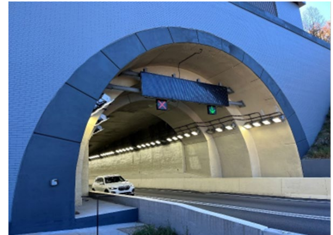
Example of a Tunnel in Bi-Directional Traffic Mode
